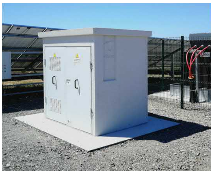
Photo 2-12: Typical cabin indoor switchgear used in the 'outdoor solar station solution' (as per Solar Station Option A)
