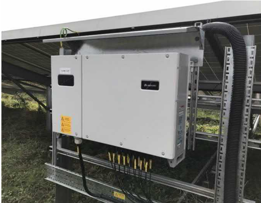
Photo 2-9: Typical string inverter ( image reproduced courtesy of Huawei )
