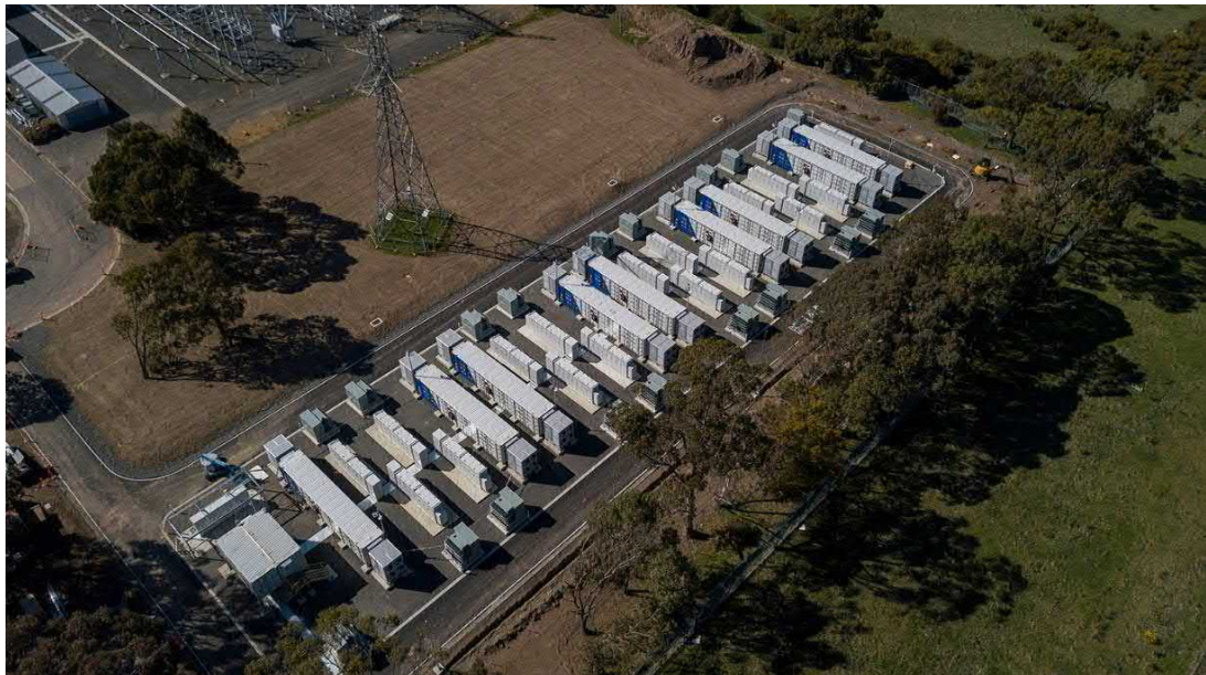
Photo 2-13: Typical battery storage compound configuration ( image reproduced courtesy of Fluence Energy )
