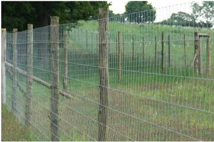
Photo 2-14: Typical deer security fence
